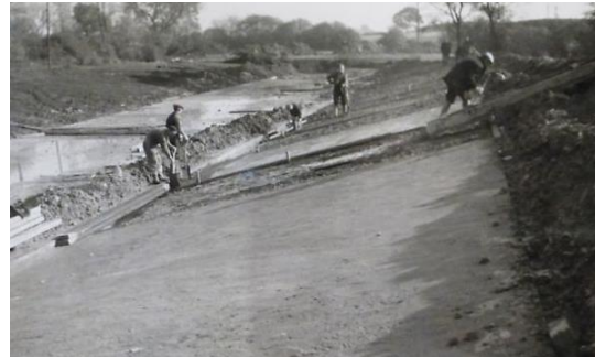
Construction on the reservoir
